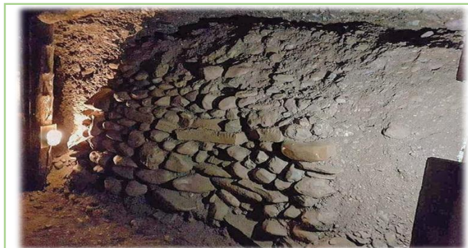
Figure 19: Large dry-stone wall in Ravne tunnel with slab and cobbled features. This dry-stone wall measures approximately 125 cm in height and 300 cm in width, making it one of the most expansive examples recorded within the Ravne Tunnel system. Constructed in twelve courses, the wall exhibits a high degree of stability and intentionality in its design. A series of horizontally embedded flat stone slabs are prominently featured in the midsection, possibly to enhance structural cohesion. Uniquely, the wall terminates at both ends with large rounded cobbles, a feature not previously observed in this form.
