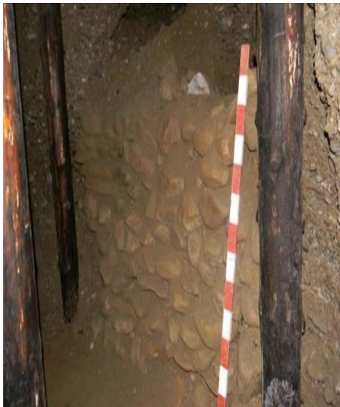
Figure 11: Dry-stone wall in the Ravne Tunnel Complex, one of over sixty discovered so far. This photo documents a typical example of the dry-stone walling technique found throughout the Ravne tunnel system. Rounded river pebbles were carefully stacked without mortar to block side passages, behind which unconsolidated fill material is typically encountered.
