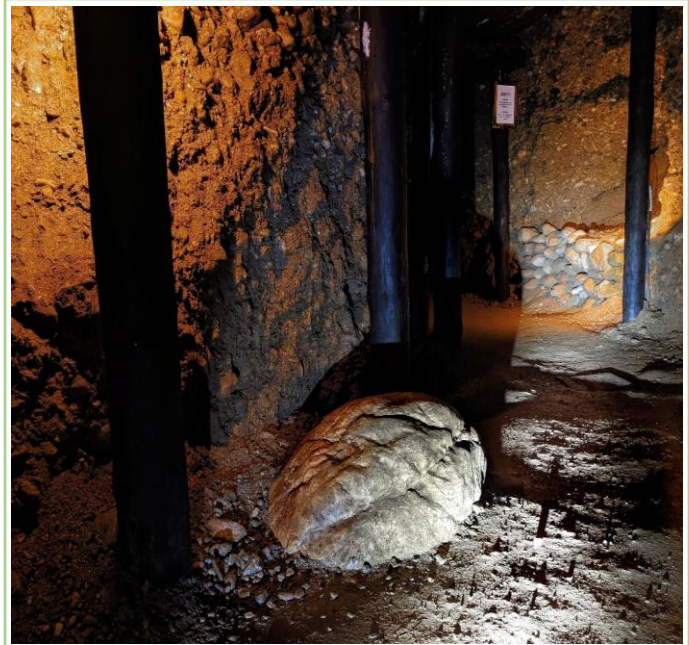
Figure 10: Tunnel segment 35 meters from the entrance to the Ravne Tunnel Complex, showing modern wooden supports and first visible dry-stone wall. This photograph captures an early section of the main Ravne tunnel where vertical wooden supports were installed by the Foundation for visitor safety. In the background, a dry-stone wall constructed from rounded river pebbles can be seen, closing off a side passage-part of a recurring architectural pattern throughout the complex. A large stone monolith is visible in the foreground, situated within the original tunnel profile [4].
