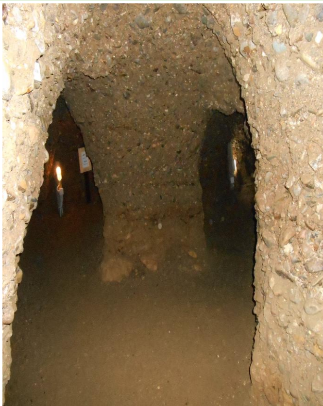
Figure 9: Tunnel intersection within the Ravne Tunnel Complex, view from main corridor toward side passages (2025). This image shows a characteristic branching point inside the Ravne tunnels, highlighting the construction geometry of intersecting passages with rounded arch-like profiles. The tunnel walls and ceiling are composed of compacted river pebble conglomerate, which remains structurally intact without artificial reinforcement. Lighting elements visible in the background mark the preserved route for visitors [12].
